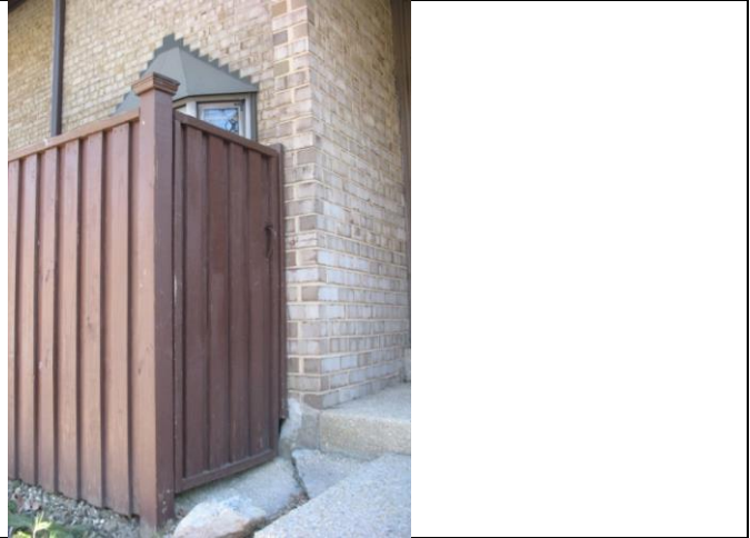
4: 9211 Gate end lag on house
